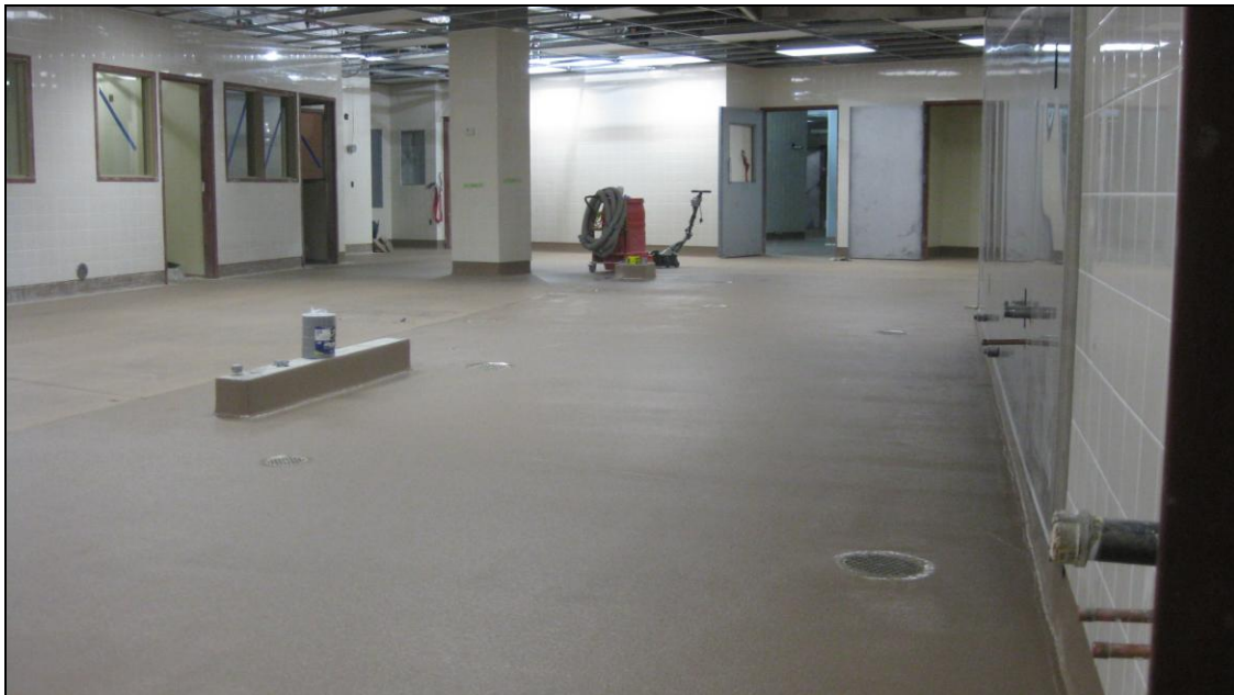
Kitchen area epoxy flooring installation
