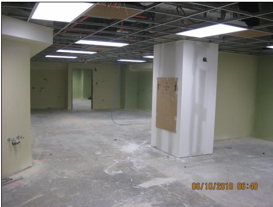
Lab progress as of June 11, 2010
