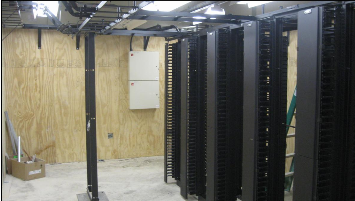
Progress in the MDF room
