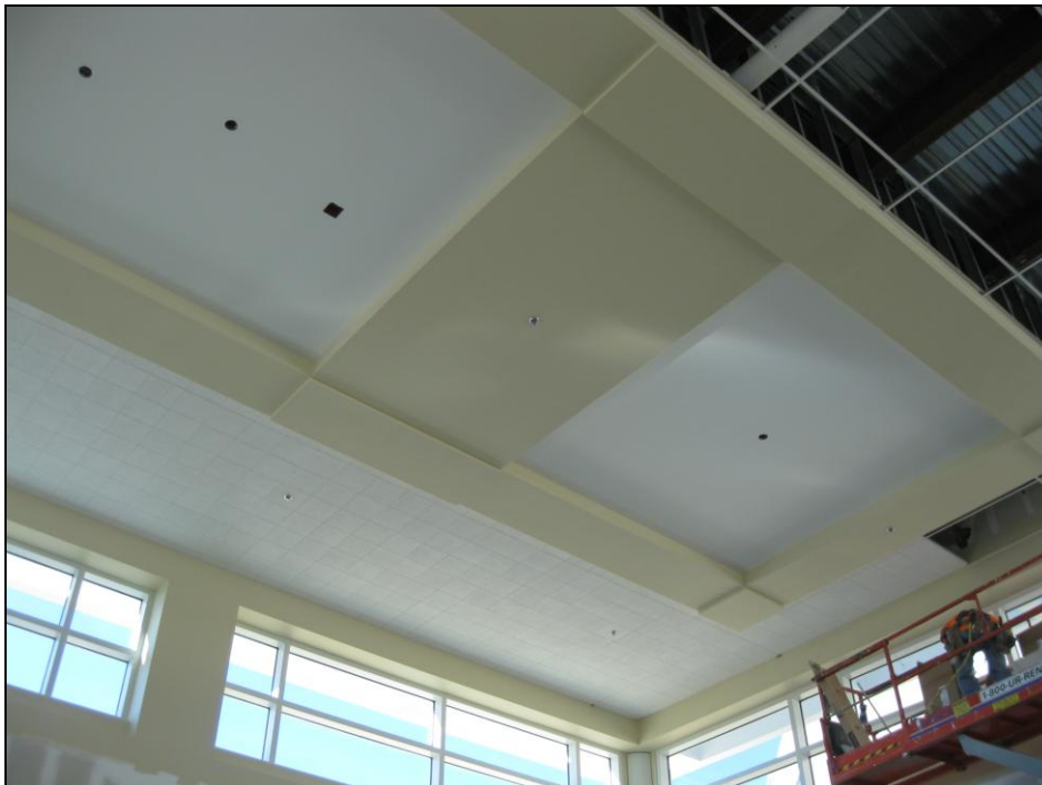
Main lobby ceiling progress
