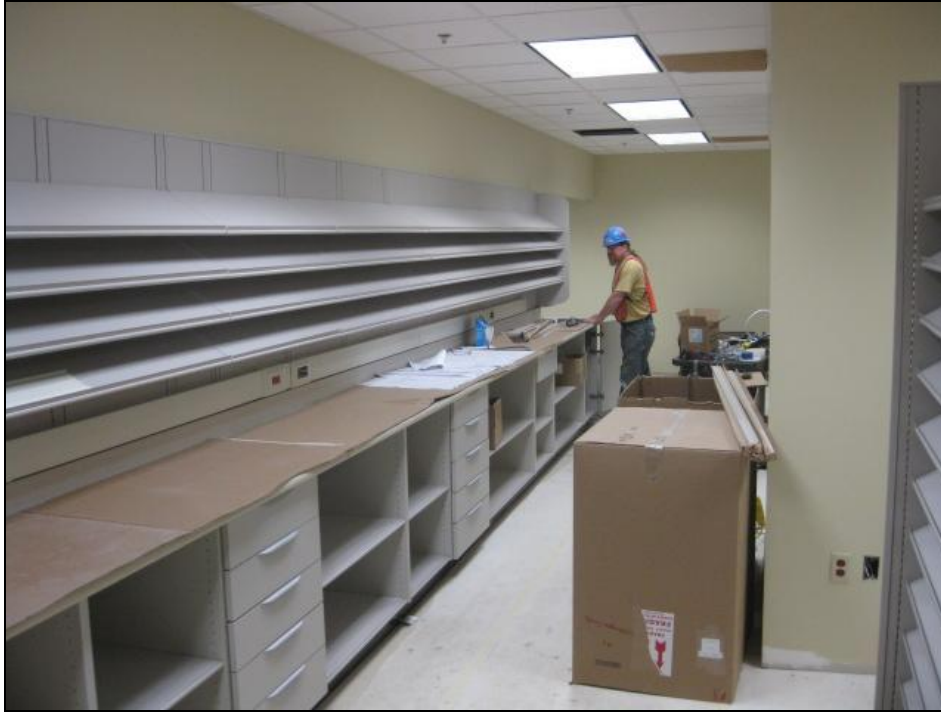
Owner Pharmacy equipment installation
