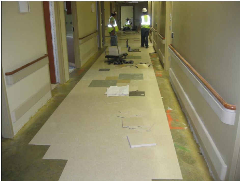
Flooring installation in LDRP
