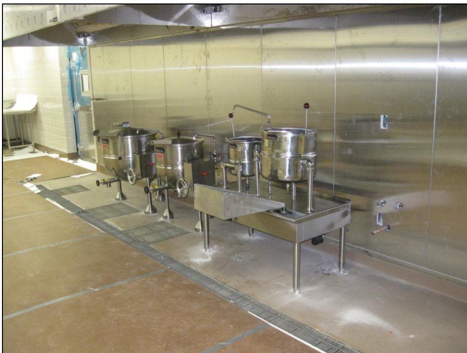
Kitchen equipment installation
